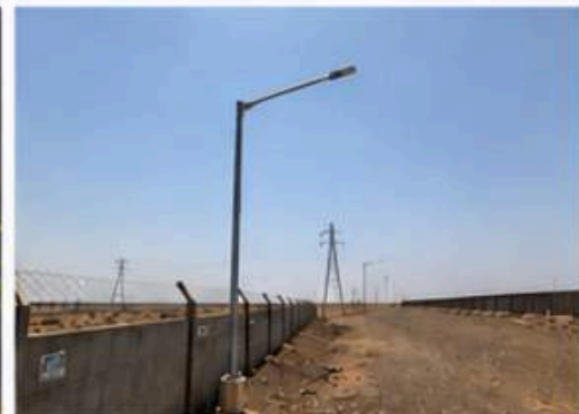
09 LED STREET LIGHT INSTALLATION
