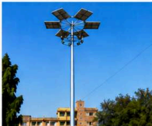
07 SOLAR HIMAST POLE INSTALLATION
